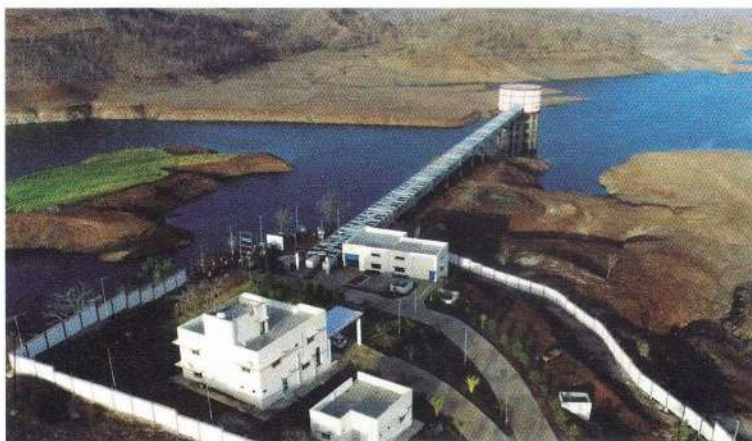
Modern engineering marvel to ensure clean tap water in every home
