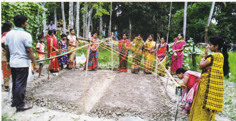
Handholding Training on Construction of Rainshelter
