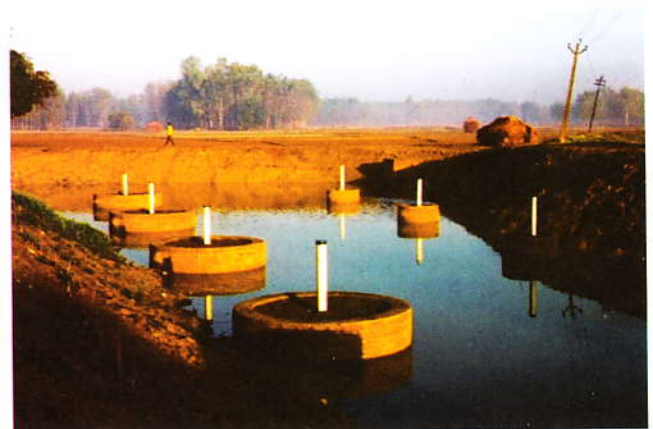
Fig. 6. An unused village pond retrofitted with UTFI technology for flood water recharge in Rampur, Uttar Pradesh
