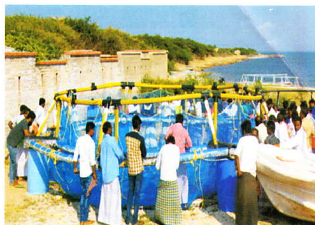
A Cage is getting ready for installation
