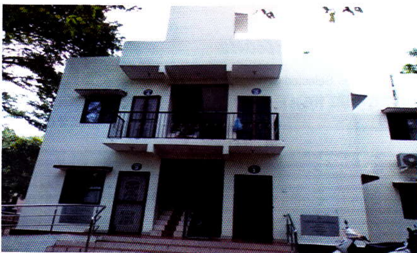
Demonstration building made of GFRG Panels in IIT Madras.
